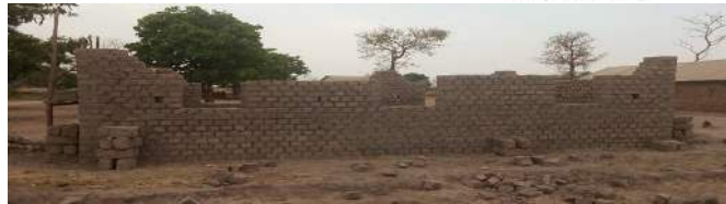
Above: Progress on building the 8m by 5m classroom for Senior 3
